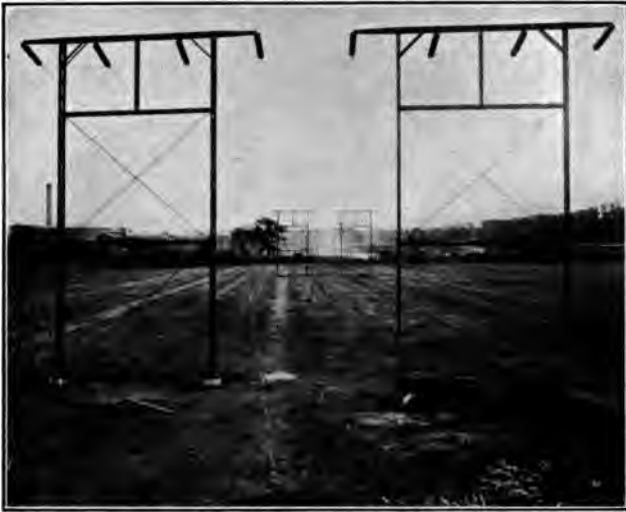
FIG. 168.—Experimental transmission line.
